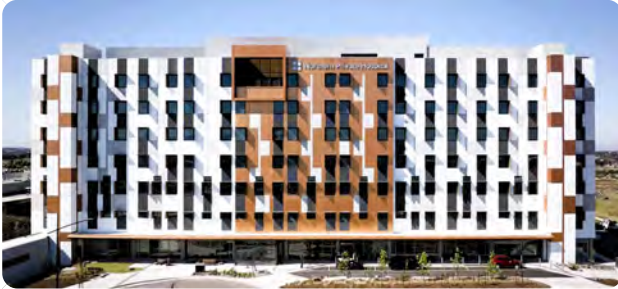
Northern Private Hospital at Epping, Victoria.
